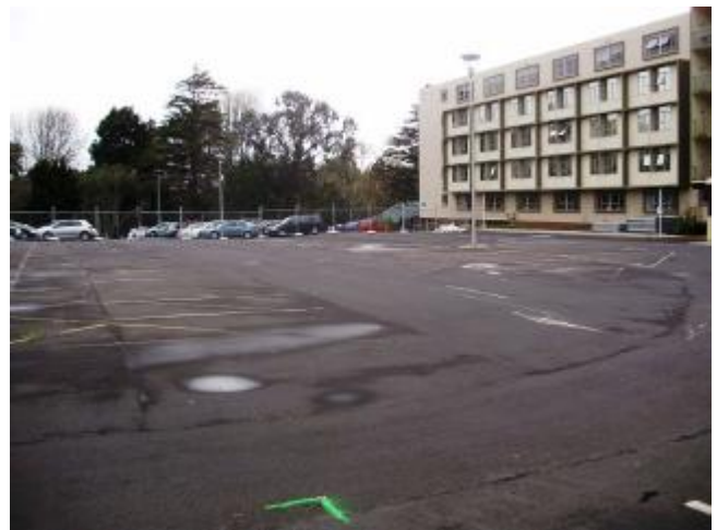
The staff car park has become a construction zone
