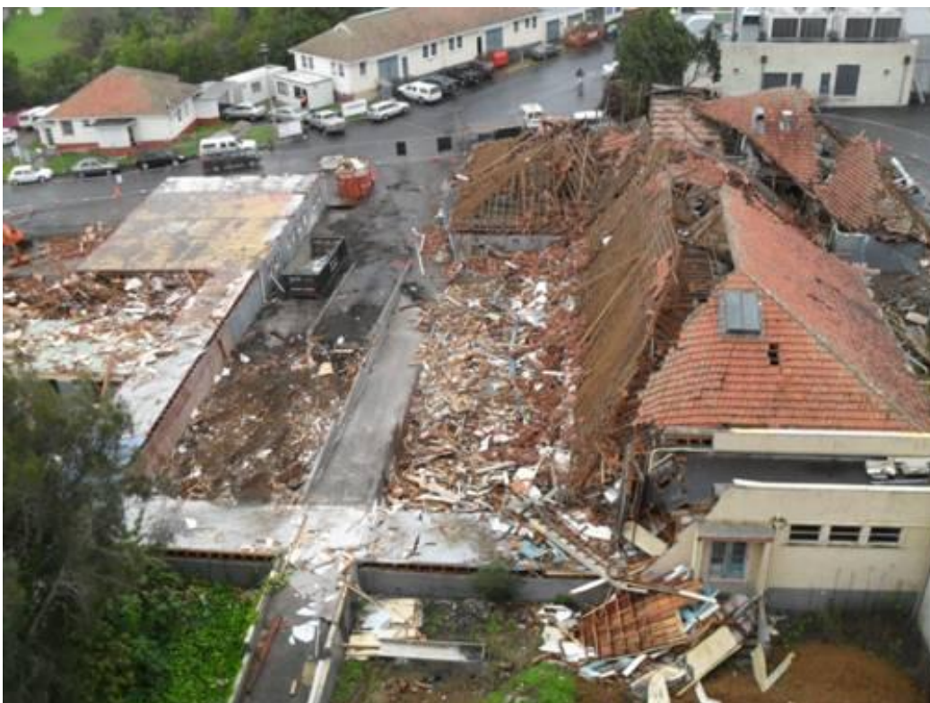
After demolition – 20 September 2010
