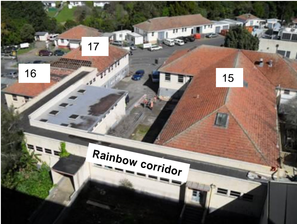
High level view of old Gastroenterology (15), Haematology (15), Linen (17), Spiritual Centre (17) and the Rainbow Corridor
