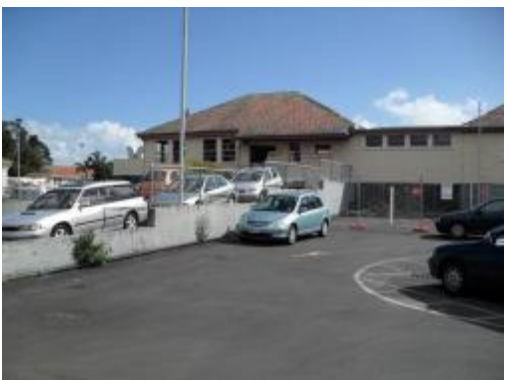
Pre-demolition: Building 17 - Linen and Groundsmen's Shed
