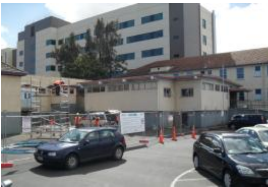
Pre-demolition: Building 16 - Clinical Coding
