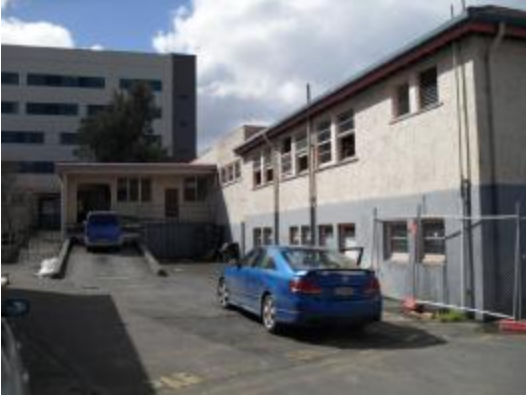
Pre-demolition: Spiritual Centre, Linen and Groundsmen's Shed
