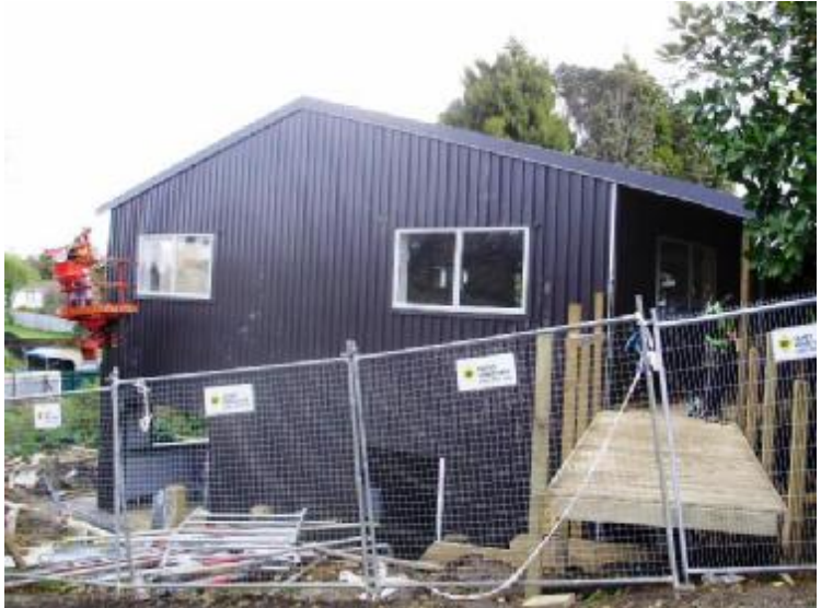
The new Building 19 is taking shape
