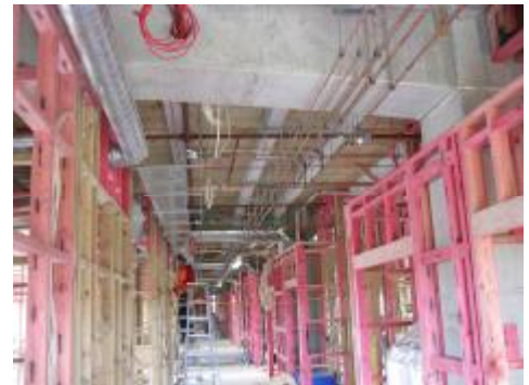
Fit-out framing is underway on Level 3.
