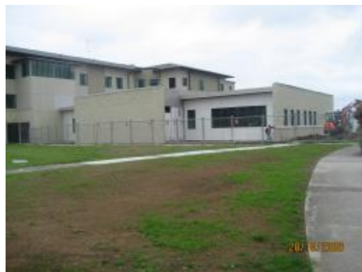
The exterior of the new Renal Unit
