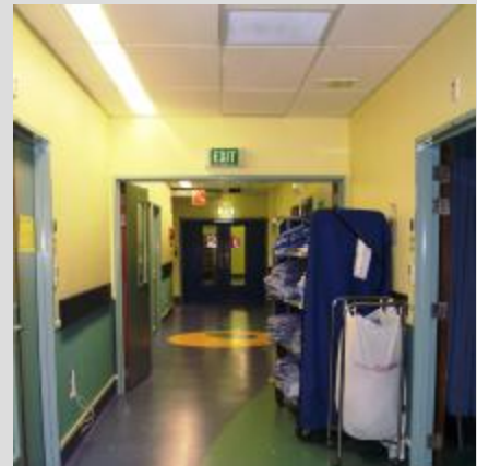
Demolition of C-Pod has begun
