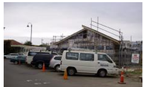
A new roof covers the expanded ward block.
