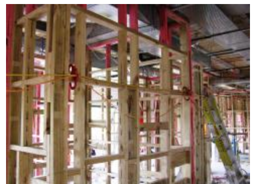
The lining of the walls will soon commence on Level 3
